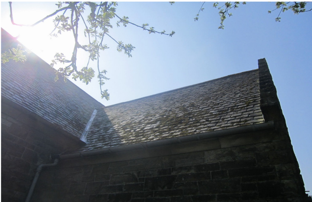
29 Moss to be removed from slate roof
