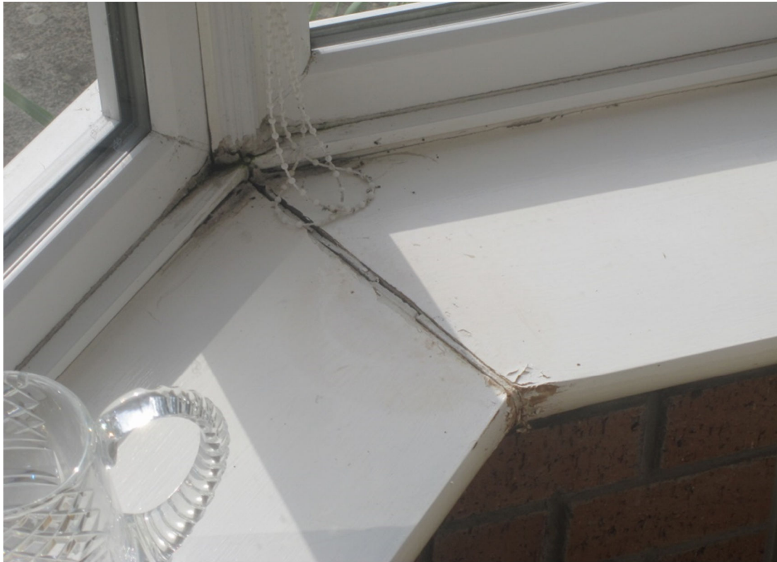
34 & 35 Open joints in window sills in conservatory
