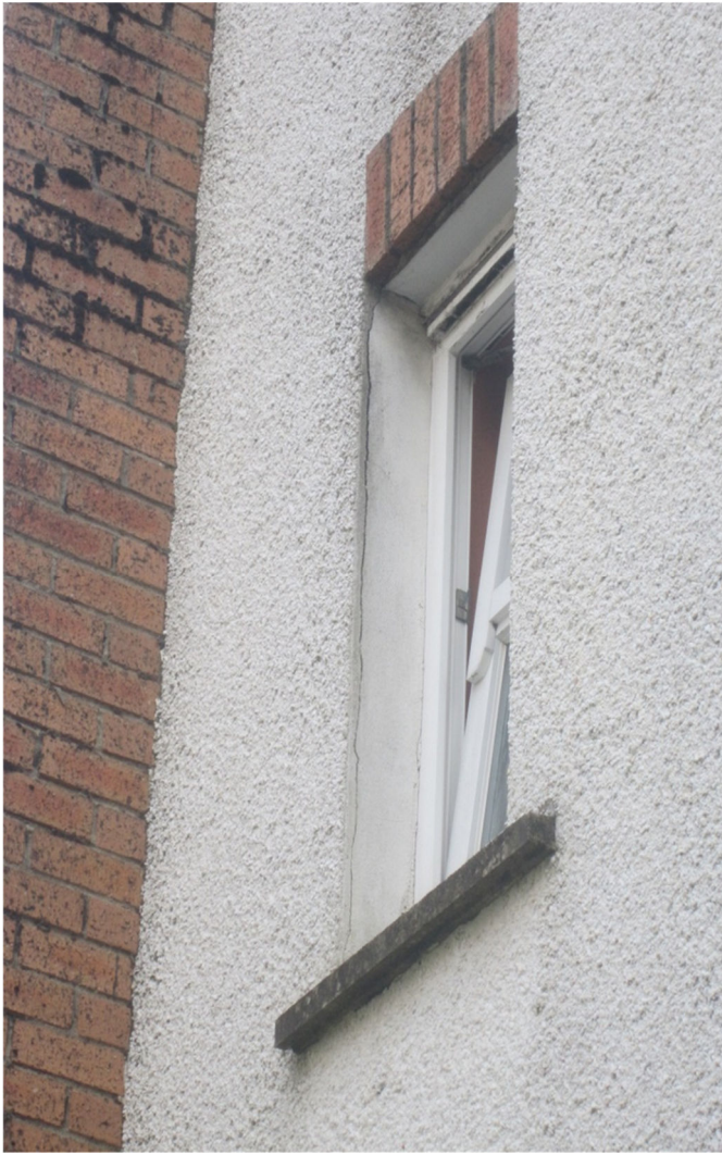
32 & 33 Render cracked at window ingoes
