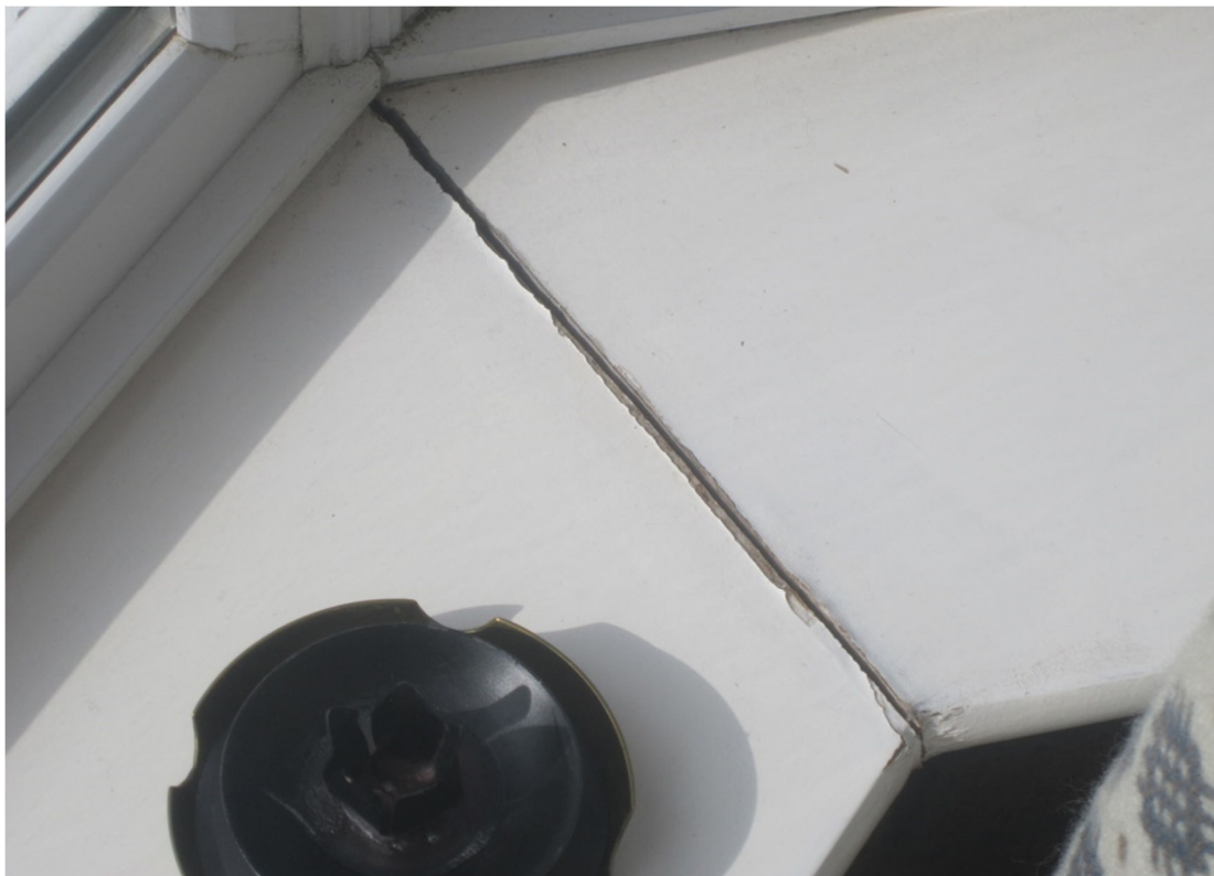
34 & 35 Open joints in window sills in conservatory
