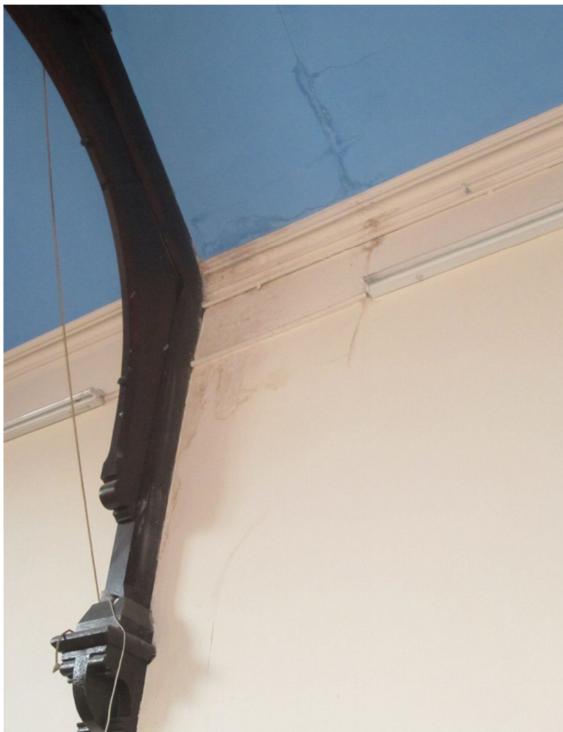
19 & 20 - Historic water ingress in large hall - plaster damaged from wifi installation
