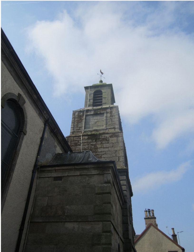
13 - Tower is mossy and has some vegetation to be removed
