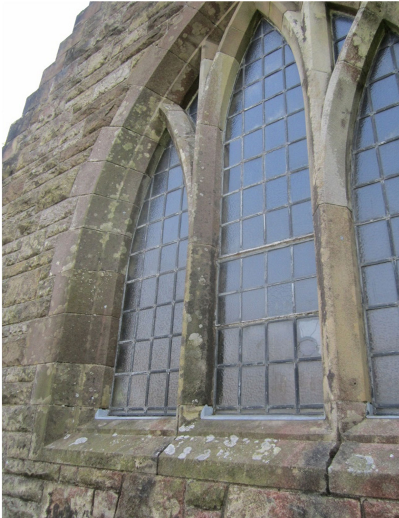
23 Open joints in ashlar stonework at window
