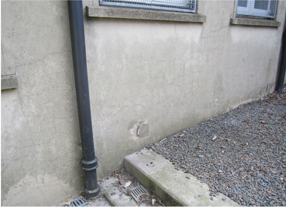
17 - Render damaged - no vents in wall
