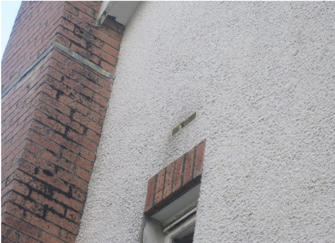
30 New grille required to vent above ensuite windows
