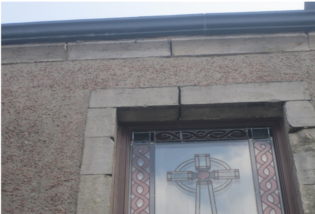
14 - Lintel above side window cracked
