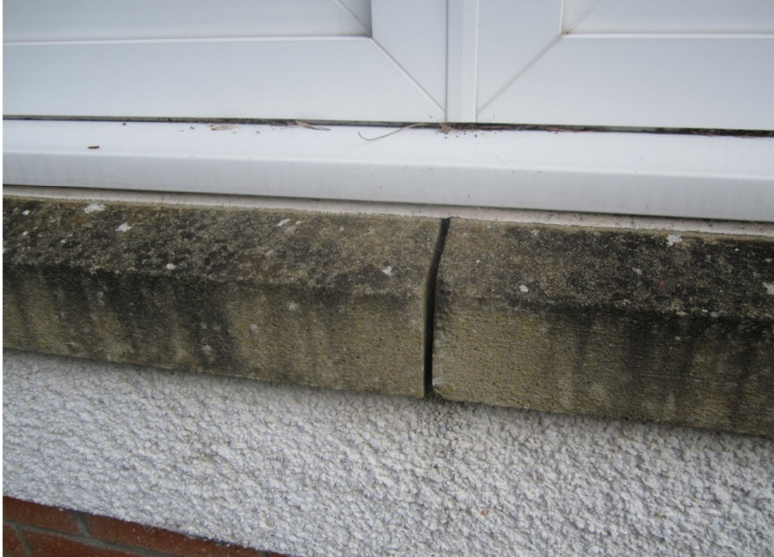
31 Open joints in reconstituted stone window sills
