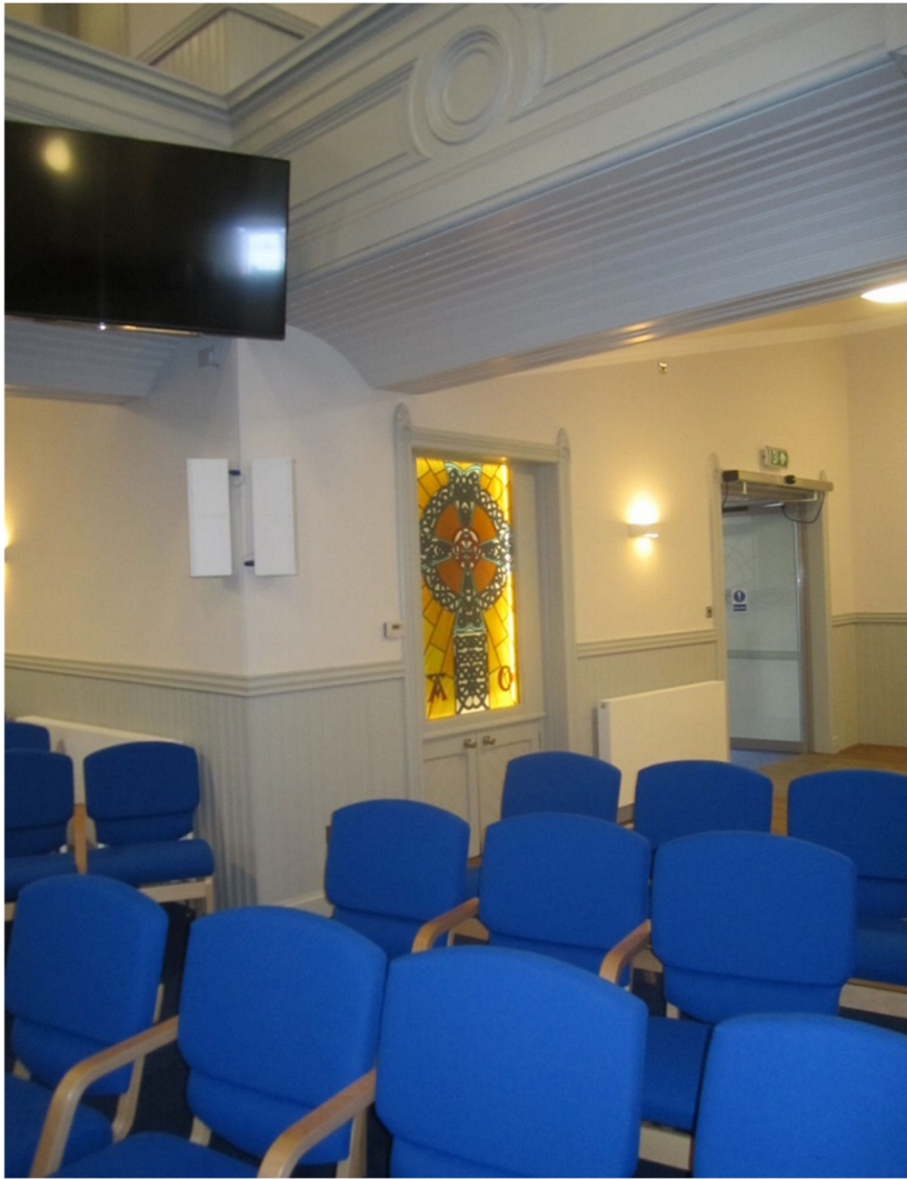
44 Door infilled and new opening with electrically operated door formed
