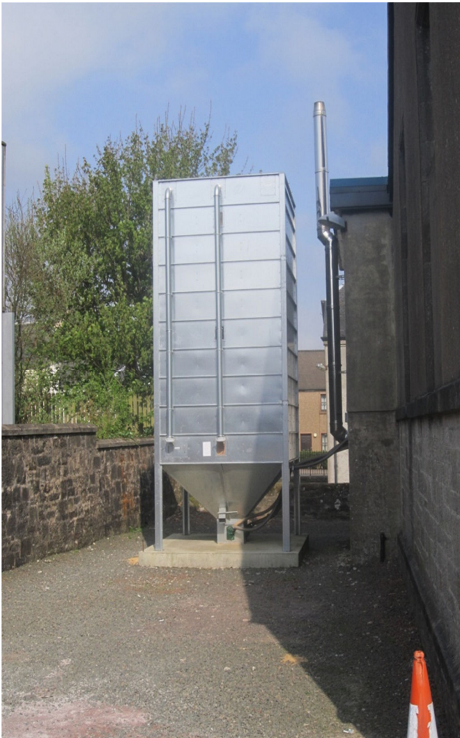
36 & 37 Biomass boiler and storage
