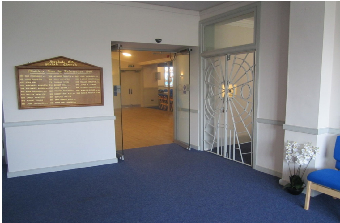
45 New electrically operated door from vestibule into sanctuary
